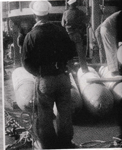
All ten of the Mark 1 Mod 2 test vehicles are being handled on the deck of the NAHANT for return to the depot.
