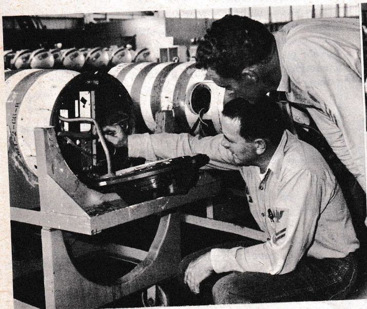
Inside, Henry and Cisco check remaining counts on ship counter for comparison with original setting . . . also visually inspect for clues to failure.
