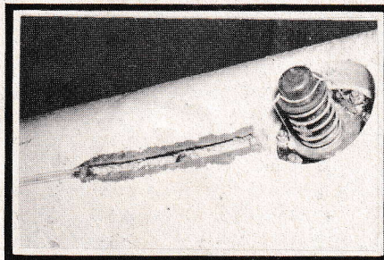
Whose weld was this? →
