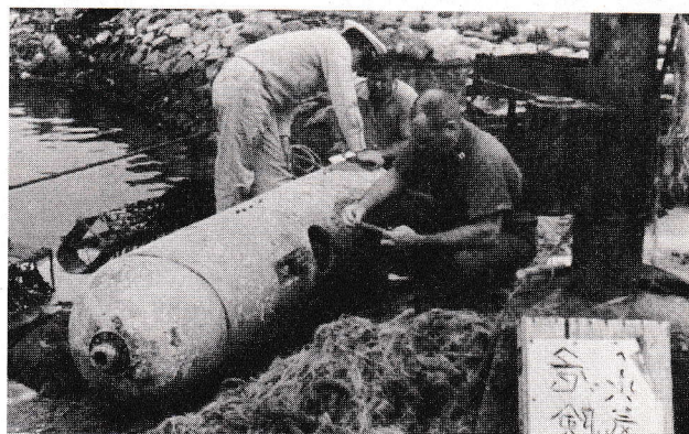
A Japanese Self Defense Force Officer looks on as BM1 W.F. Lackey (left) and LT J.D. Connor, Explosive Ordnance Disposal men, disarm explosive loaded Mk 12 mine.
